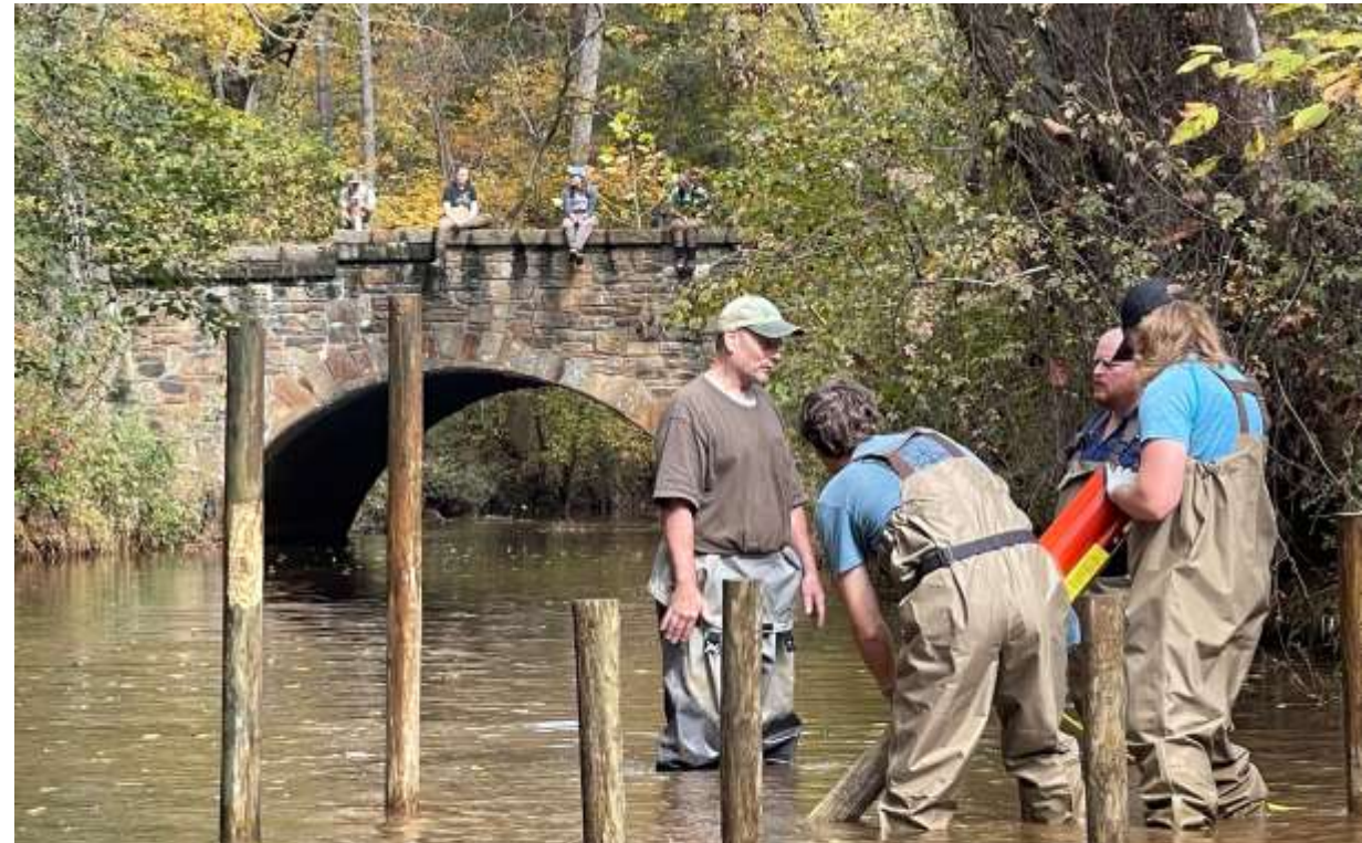
Daniel Hanks and others install posts for habitat enhancement, 2023.
