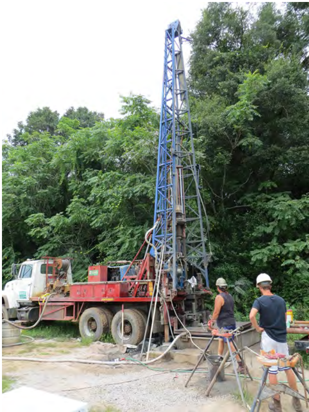
Figure 19. USGS drillers collecting core samples from the Creston site in Calhoun County in July 2013.
