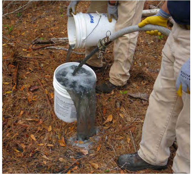
Figure 30. Before installing ADR equipment into the Dixie Plantation well, the well was pumped to flush out stagnate water and sediment that may have accumulated in the well during the years since it had been used.
