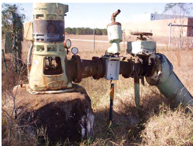
Figure 12. This unused industrial well (ORG-0079) in central Orangeburg County was added to the network in 2010 to monitor the Middendorf aquifer.
