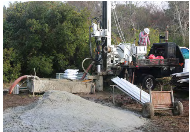
Figure 26. Drilling the two new wells at Garris Landing in Charleston County.
