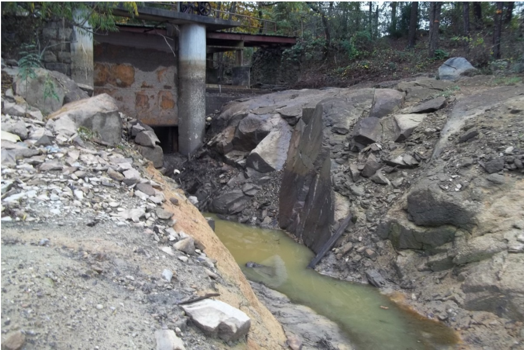
Photo 12: View shows the mill race bypass channel.
