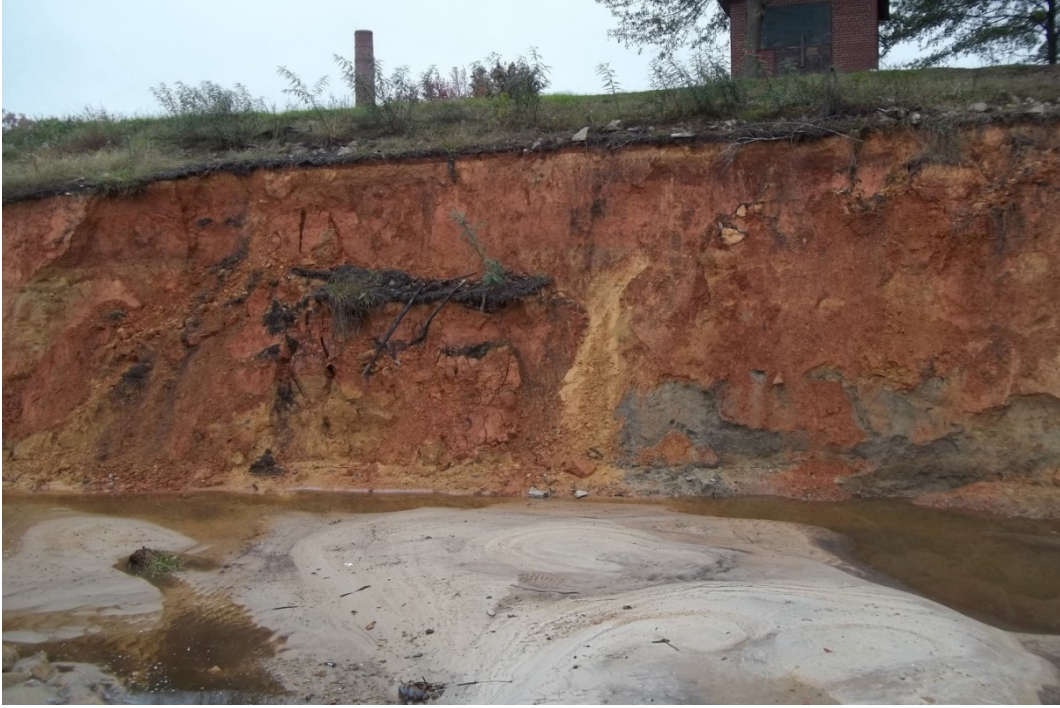
Photo 9: View is looking at upstream face of dam.
