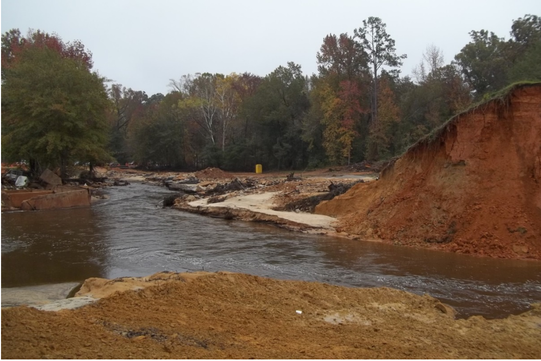
Photo 19: View is looking downstream at dam breach.
