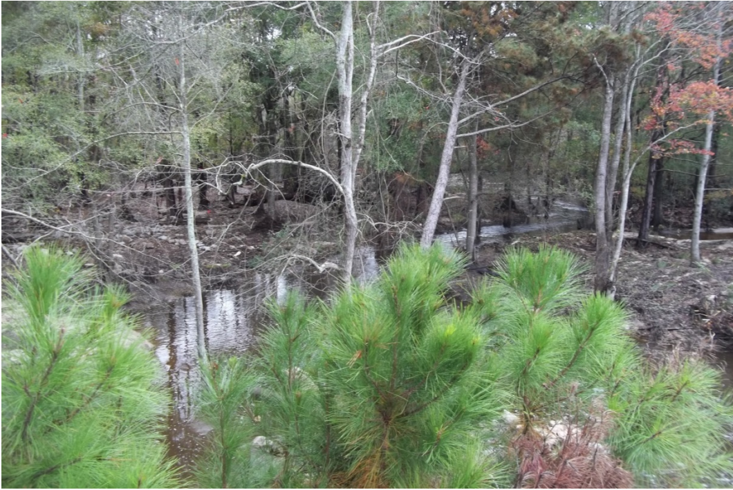
Photo 4: Looking downstream from top of dam.
