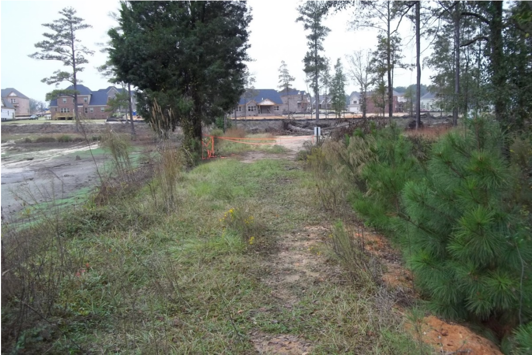
Photo 1: Left abutment on top of dam.
