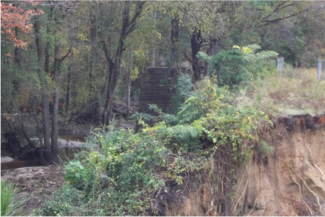
Photo 6: 28-foot concrete gate structure.
