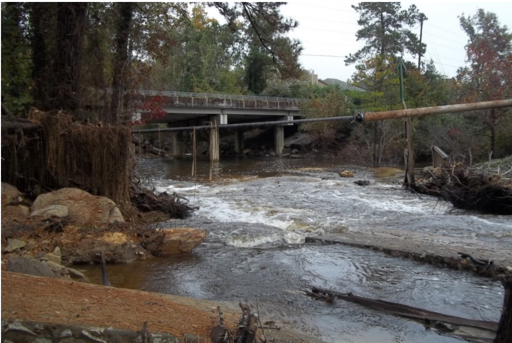
Photo 2: View from approximate dam centerline looking downstream.
