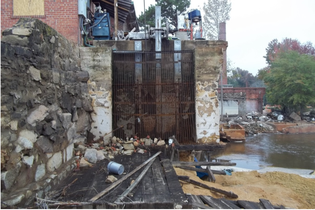
Photo 15: View is at left abutment sluice gate looking downstream.
