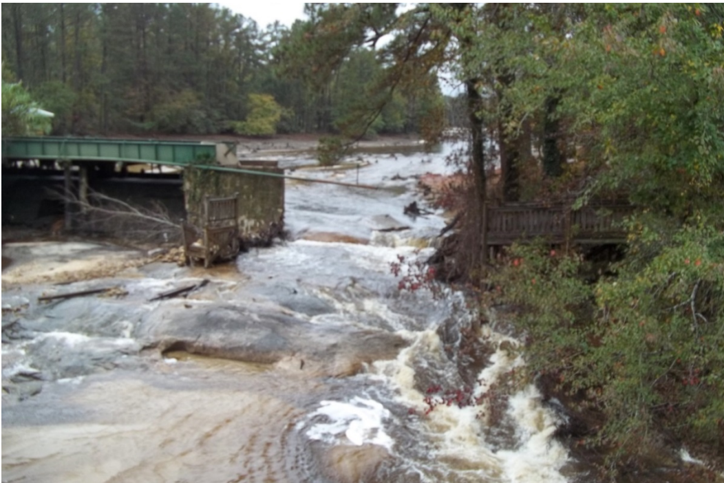
Photo 6: Looking from Gibson Road Bridge at left abutment.
