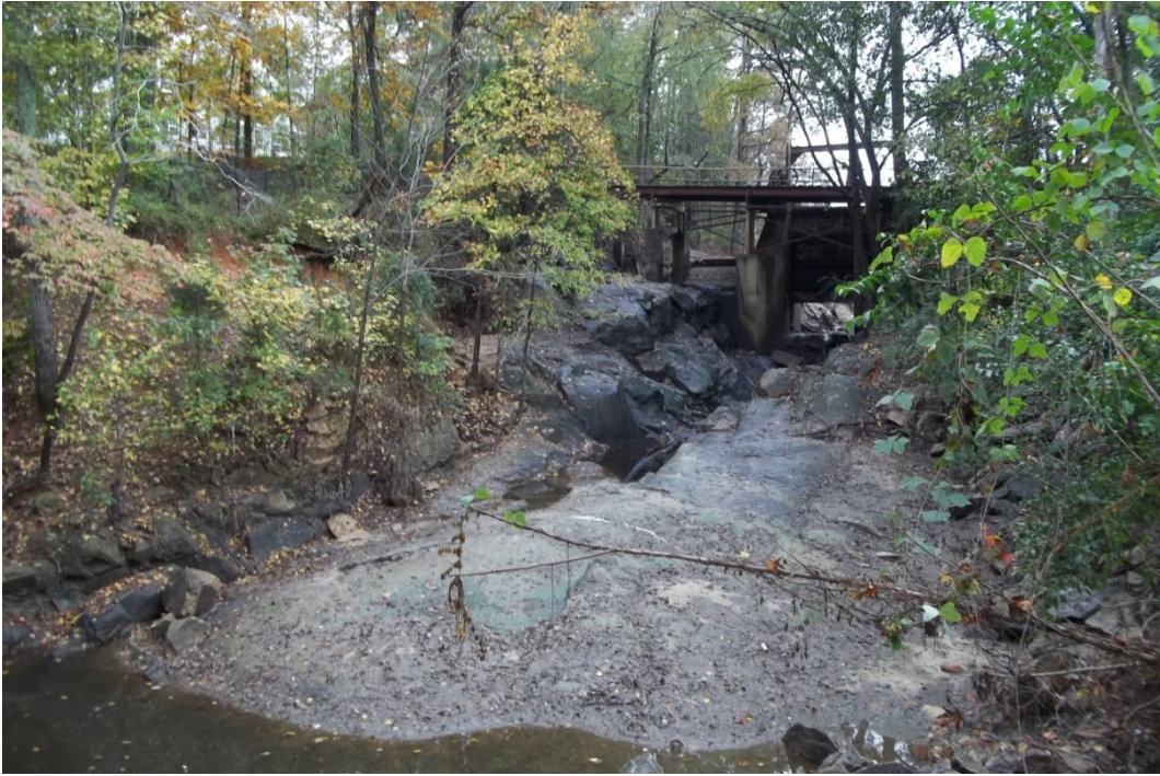
Photo 14: View is looking at downstream face of mill race bypass channel.
