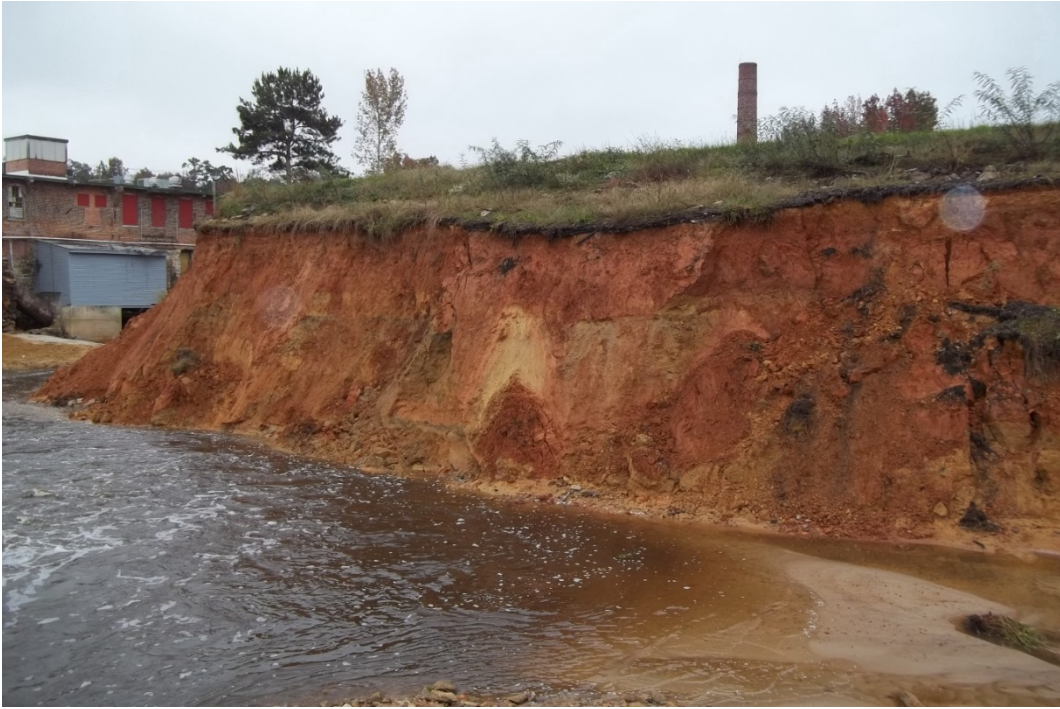
Photo 10: View is looking at upstream face of dam.
