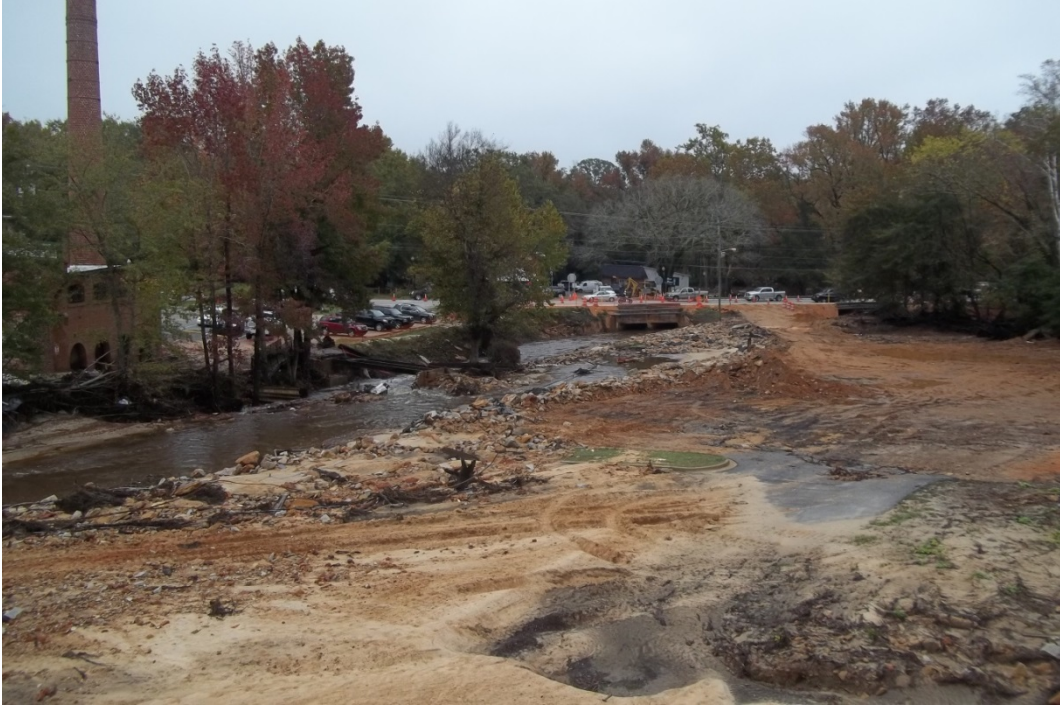
Photo 13: View is from standing on right abutment looking downstream.
