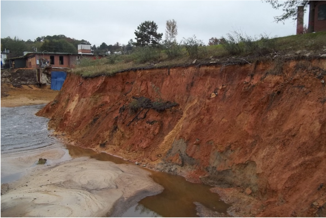
Photo 6: View is looking at upstream face of dam.
