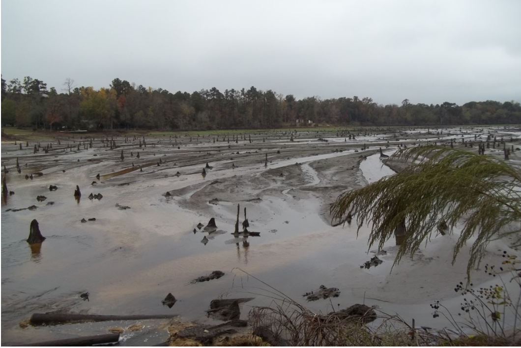
Photo 3: Looking upstream from top of dam.
