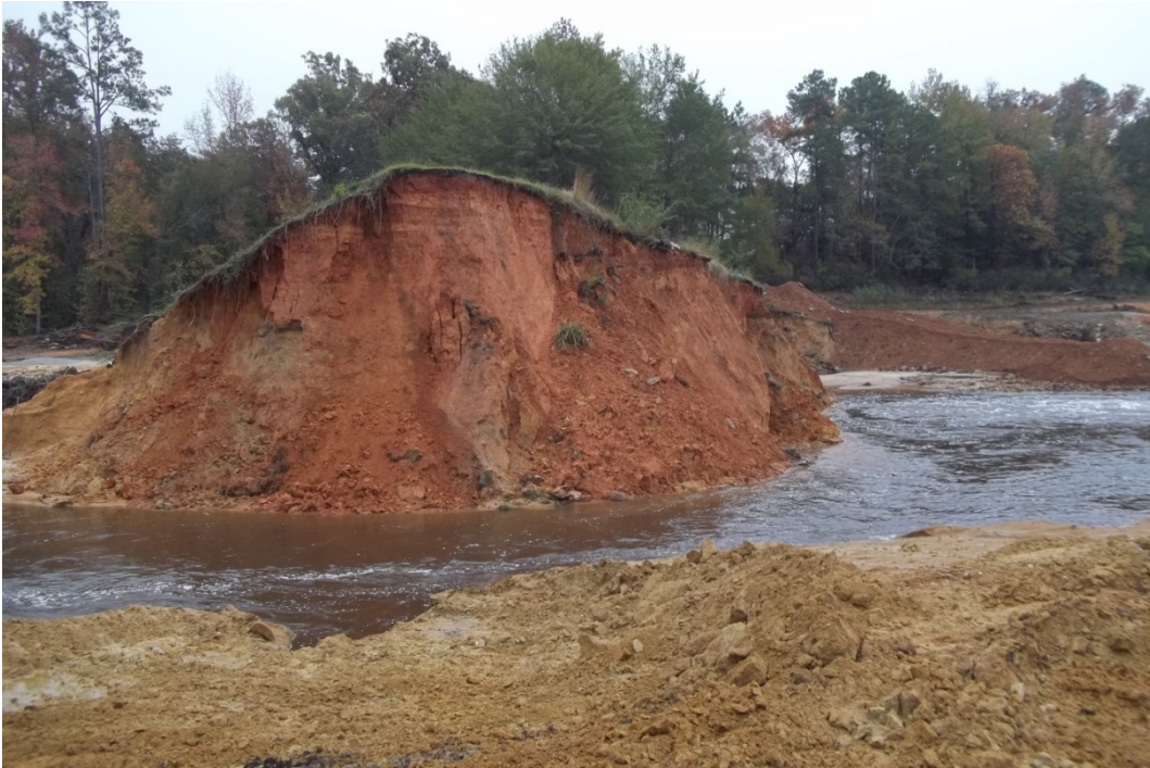
Photo 18: View is looking at dam breach from left abutment.
