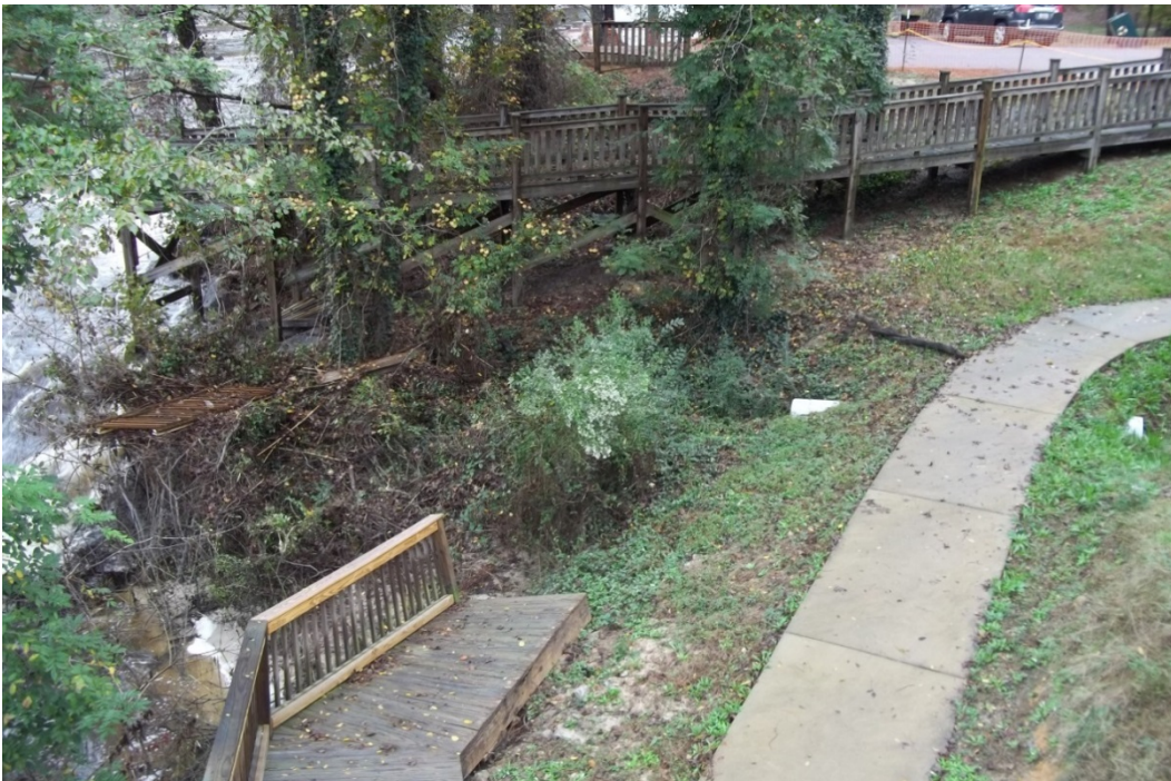
Photo 8: Wooden observation deck piers and walkway on left abutment.
