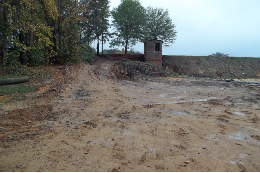
Photo 3: View shows downstream face of right abutment
