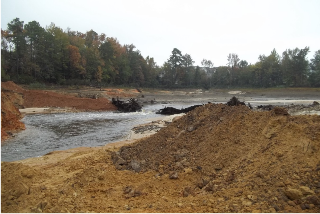
Photo 16: View is looking upstream from left abutment.
