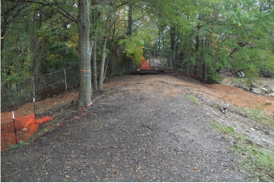
Photo 5: View is from top of dam looking at right abutment.
