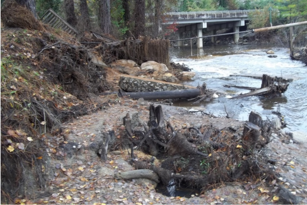
Photo 1: Left abutment looking downstream.
