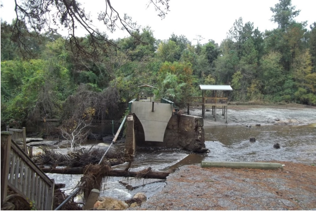
Photo 5: View from left abutment along centerline of dam.
