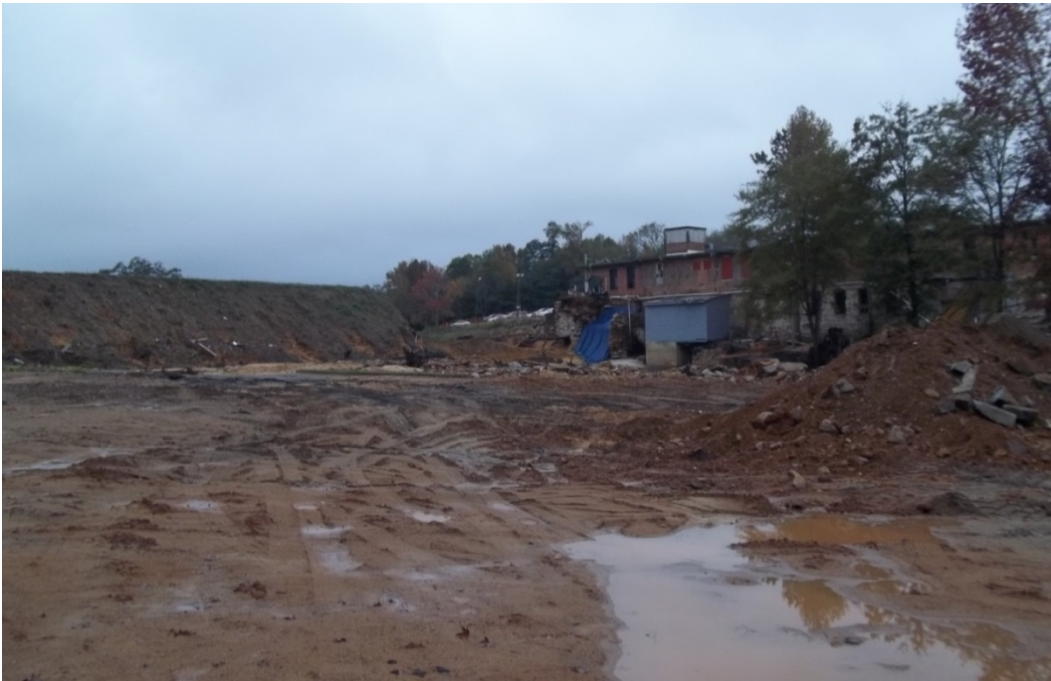
Photo 2: View is looking at downstream face of dam left abutment.
