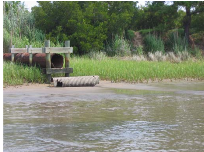
Figure F-8. Additional spoil area outfall located in Area 06B.
