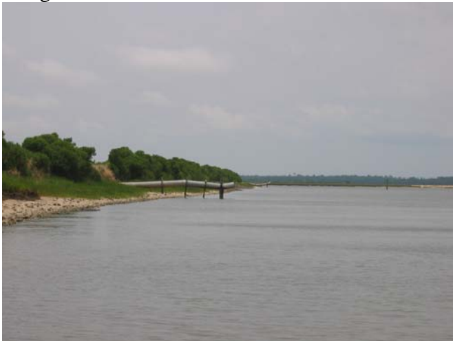
Figure F-7. Additional outfall in same spoil area as figure F-5.
