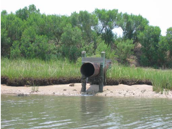
Figure F-5. Dredge Spoil Area outfall on AIWW North of Harbor River.
