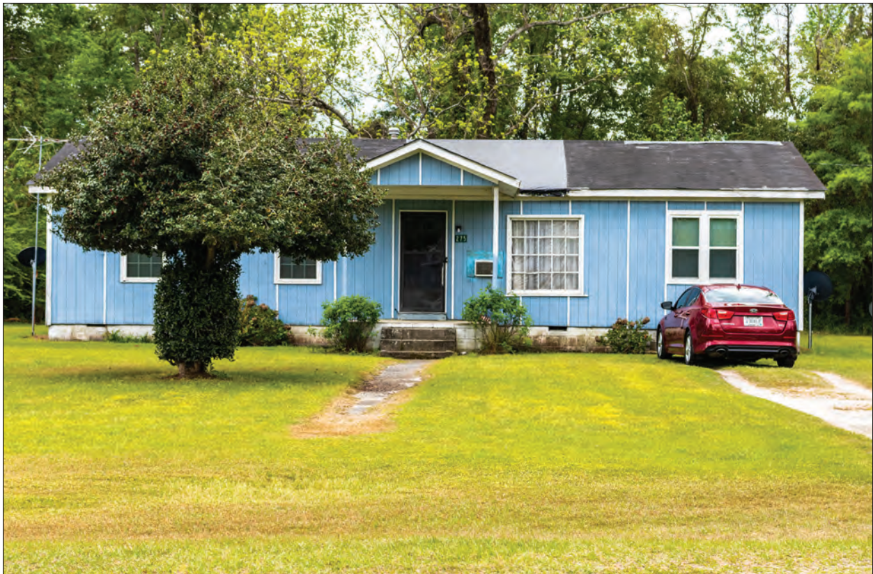
Figure 3.11 SHPO Site No. 0401, north elevation, facing south.
