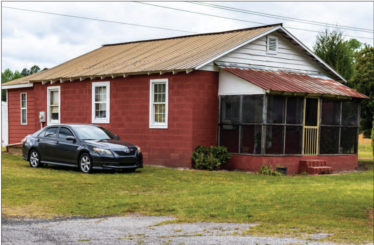
Figure 3.9 SHPO Site No. 0399, east oblique, facing west.
