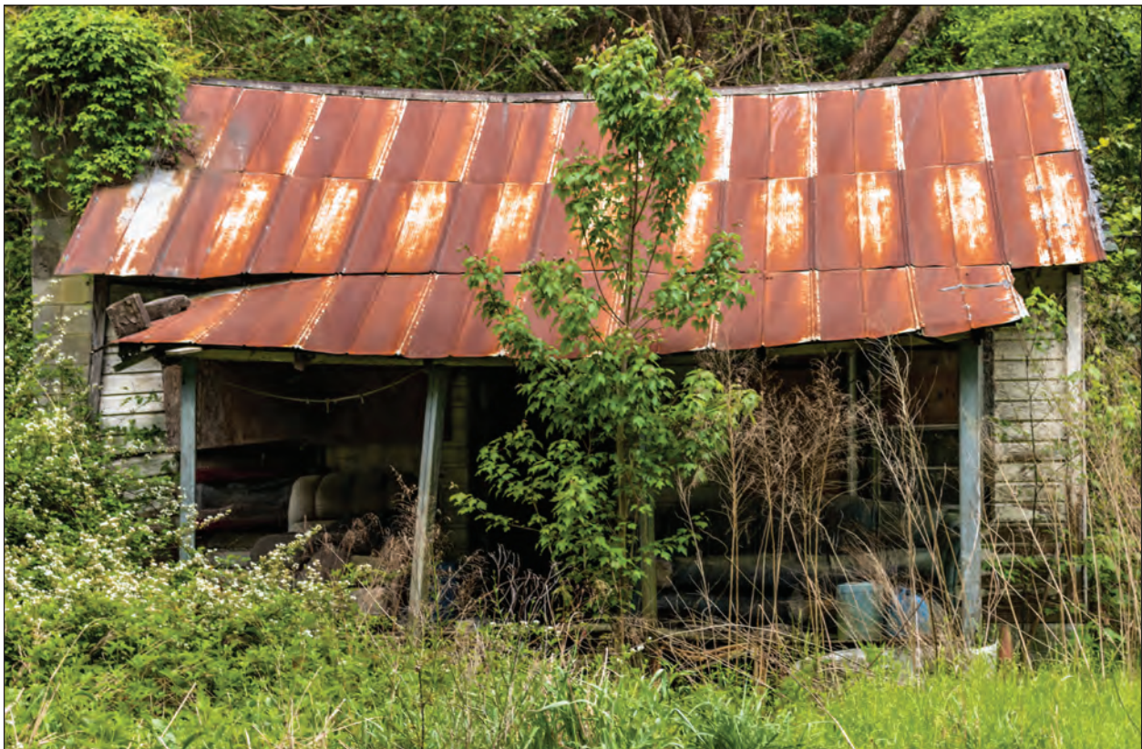
Figure 3.10 SHPO Site No. 0400, northeast elevation, facing southwest.
