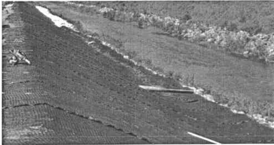
PHOTOGRAPH 3-2 INSTALLATION OF EROSION PROTECTION MAT ALONG CHANNEL SLOPE
