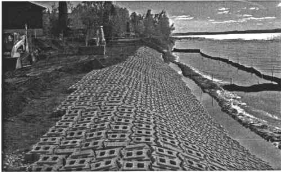
PHOTOGRAPH 3-1 INSTALLATION OF ACBs ALONG SHORELINE
